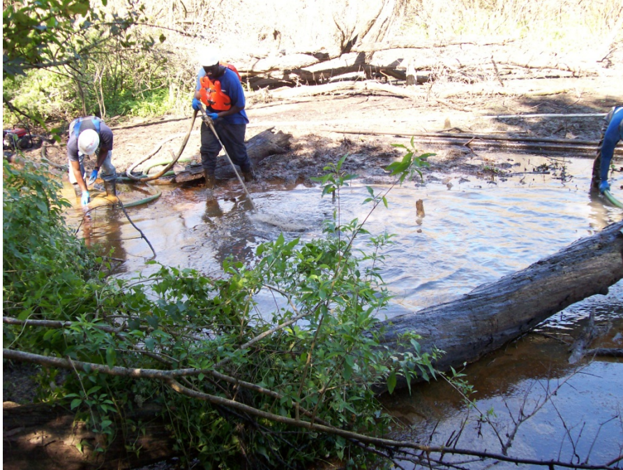
Utilizing Wash Pumps to Flush the Area of Crude Oil in Zone 1
