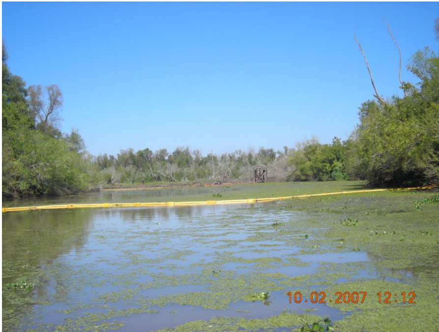
Containment Boom being utilized at the perimeter of Zone 1
