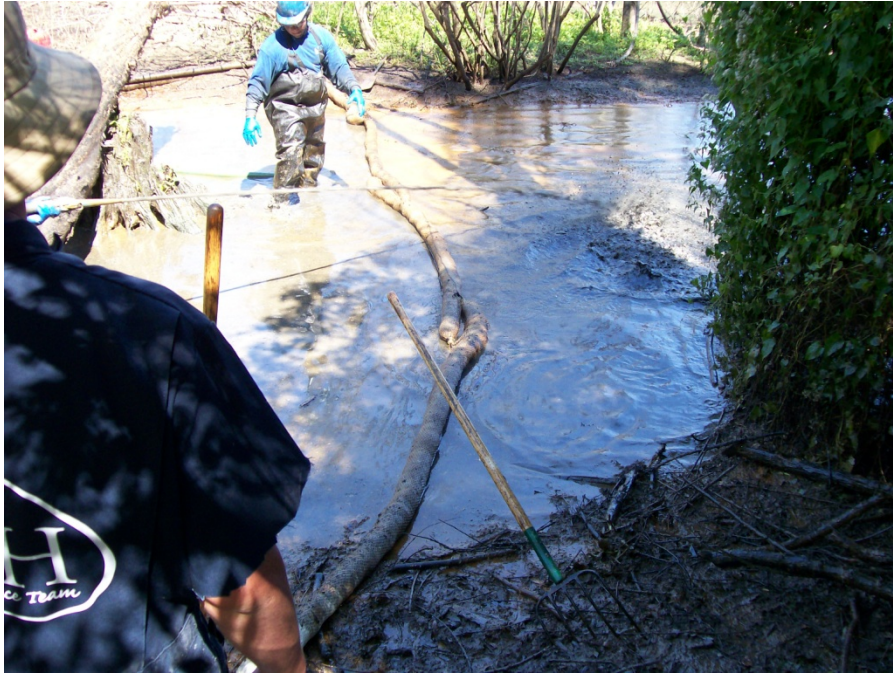
Utilization of Absorbent Boom for Crude Oil Removal in Zone 1
